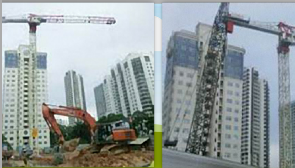
ST THOMAS WALK (TC1) JOB SITE , SINGAPORE PROJECT
