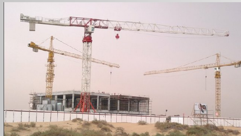
SHARJAH PRIVATE SCHOOL BUILDING
