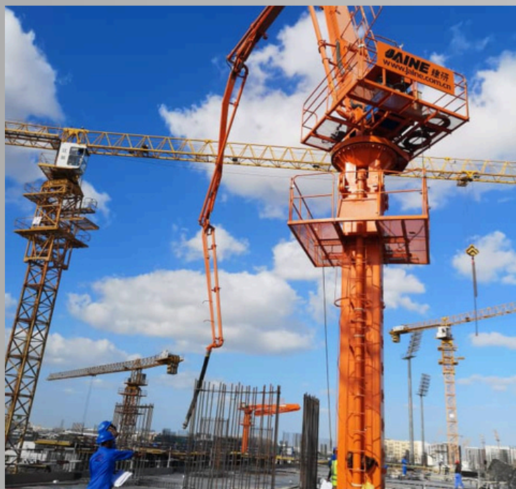
Concrete Placing Booms
