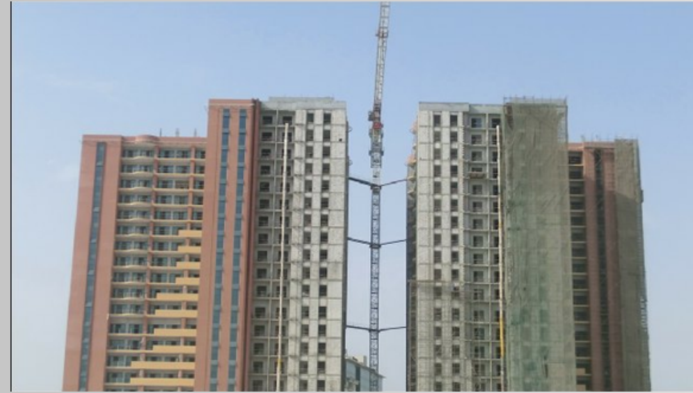
MAMZAR RESIDENTIAL TOWER
