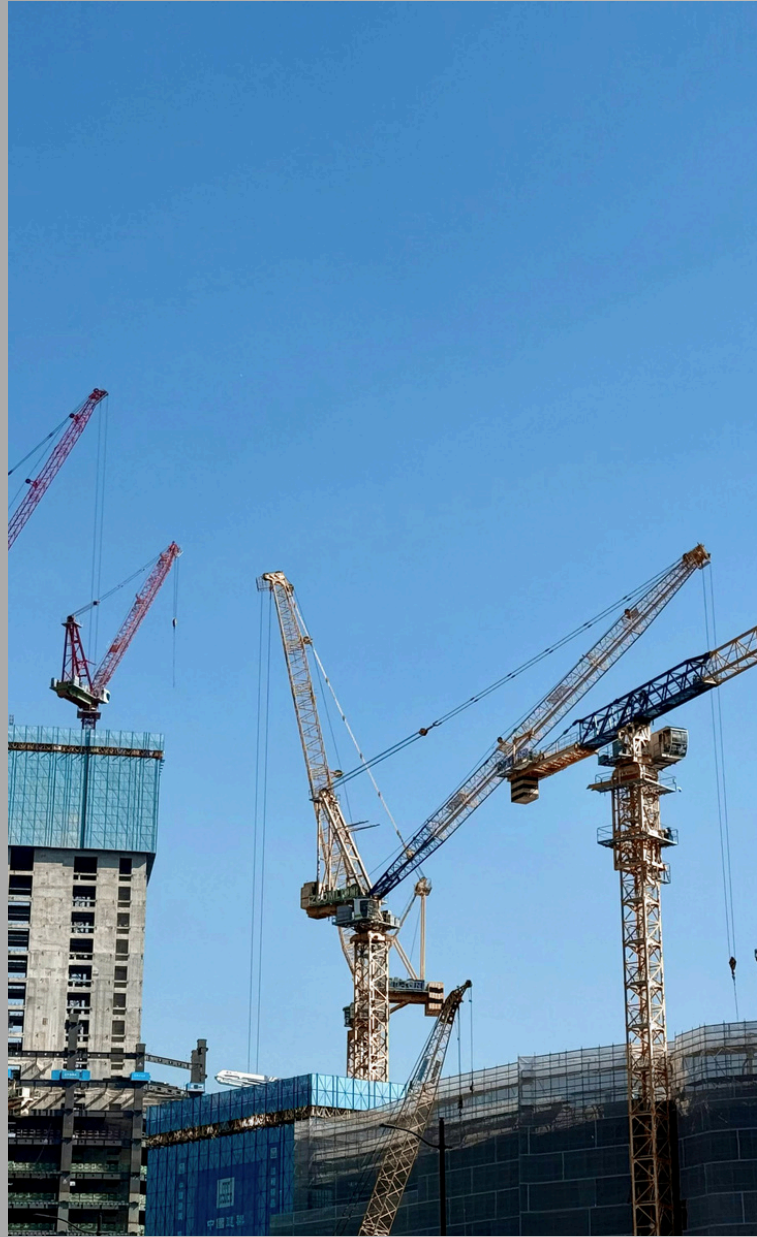
Self Erecting Tower Cranes
